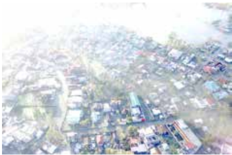
Aerial photo shows the aftermath of Typhoon Ulysses along Camarines Sur. President Rodrigo Roa Duterte conducted aerial inspections of severely affected areas in Cagayan Valley and Bicol Region on November 15, 2020. Rey Baniquet, Presidential Photo
