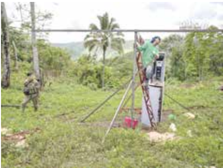
Contractors installing a water pump in Padas, in the Philippines, on April 13, 2019.
