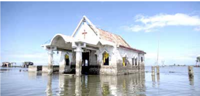
This photo taken on January 11, 2019 shows a chapel amid encroaching bay waters in Sitio Pariahan, Bulacan. Areas north of Manila like the provinces of Pampanga and Bulacan have sunk four-six centimetres (1.5-2.4 inches) a year since 2003, according to satellite monitoring. The creeping bay waters put people and property at risk, while the threat is amplified by high-tides and flooding brought by the roughly 20 storms that pound the archipelago every year.
