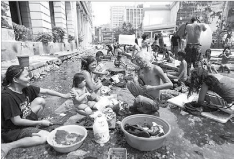
‘FREE WATER’ IN DOWNTOWN MANILA – Residents turn part of downtown Manila into their own bathroom as they make the most of free water coming from a leaking pipe in Plaza Lacson, Sta. Cruz, Manila, yesterday. (Michael Varcas)
